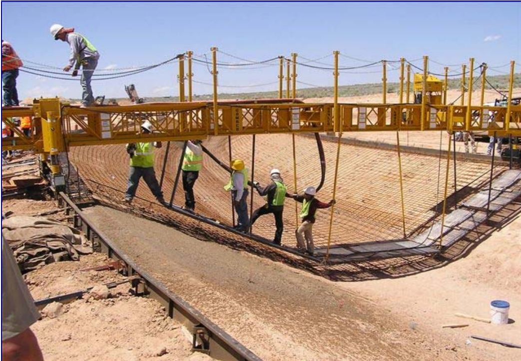
East branch of the Cabezon Channel in Rio Rancho under construction.
