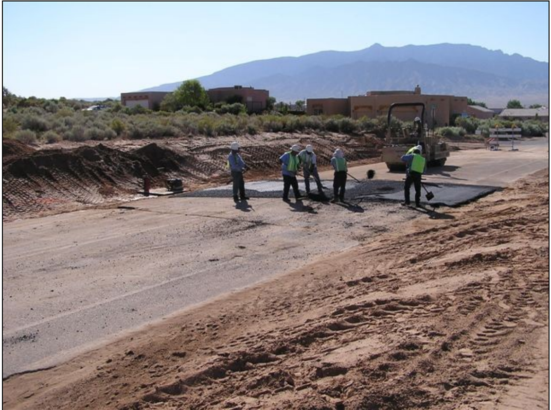
Repaving Obregon Road in July 2005
