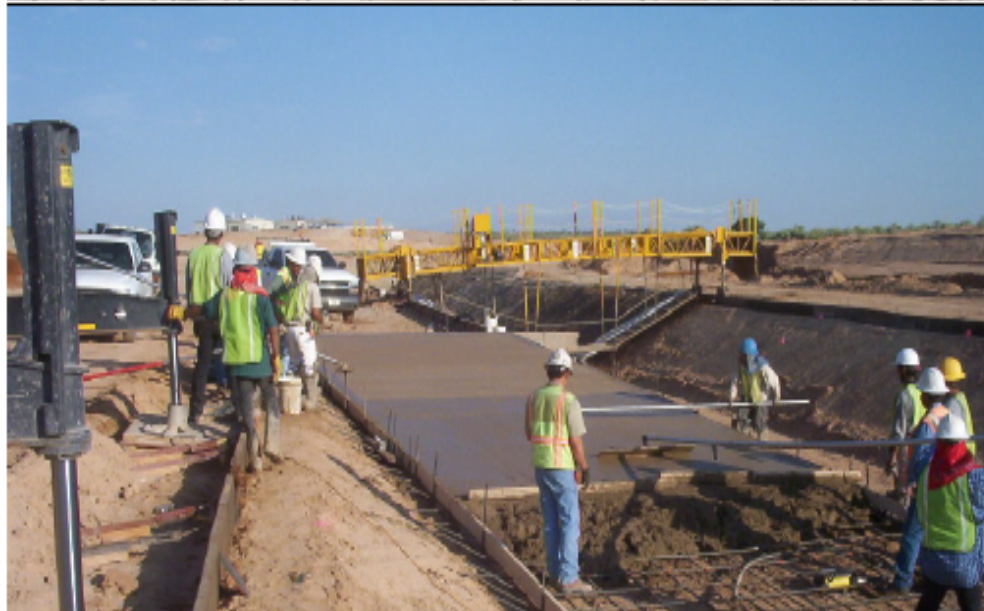
Work continued on the east branch of the Cabezon Channel.
