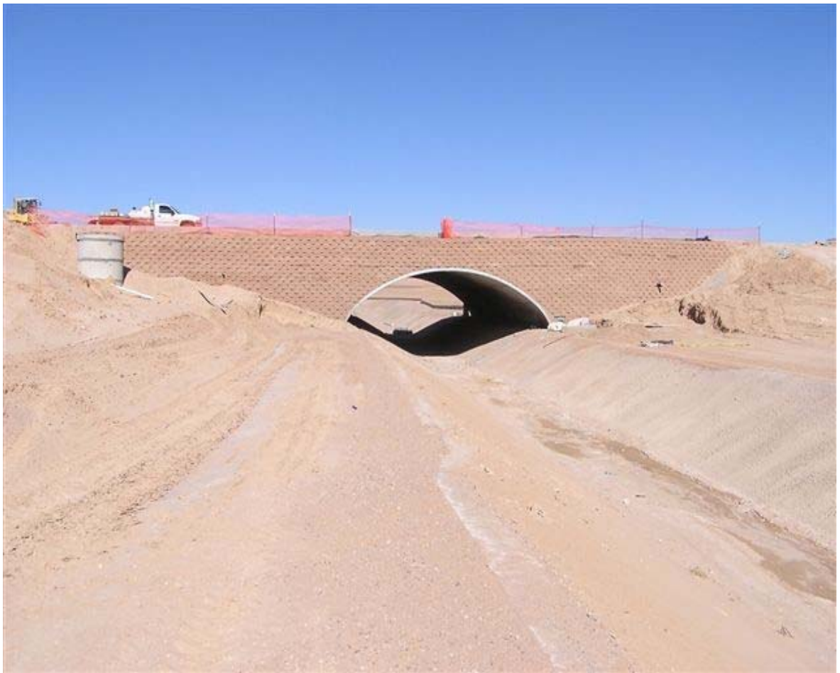
The completed Multi-Plate in December 2005
