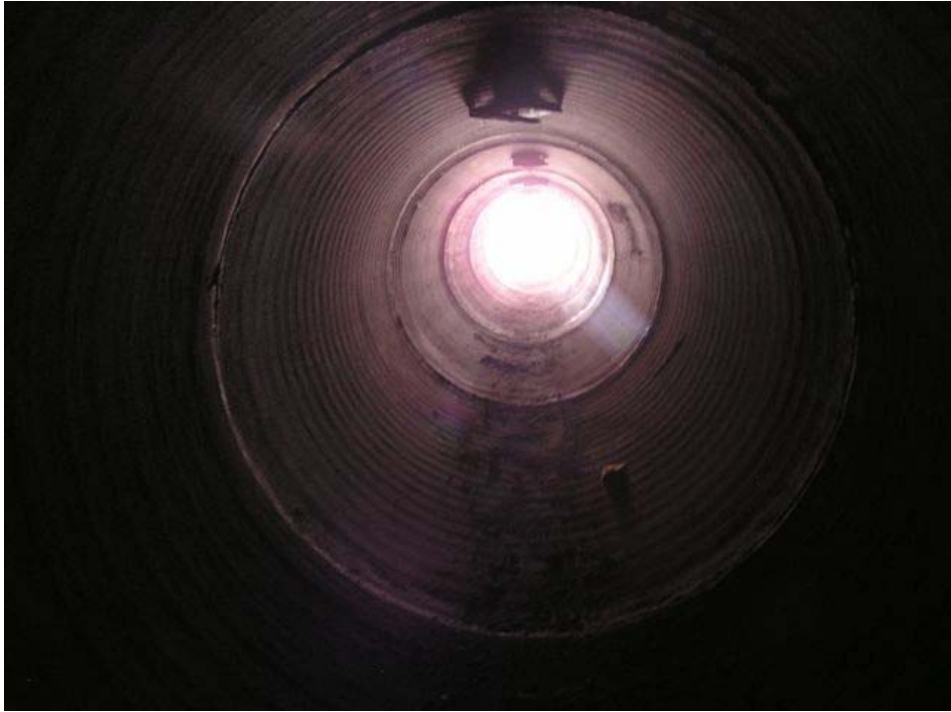
Inside the culvert being installed on Obregon Road
