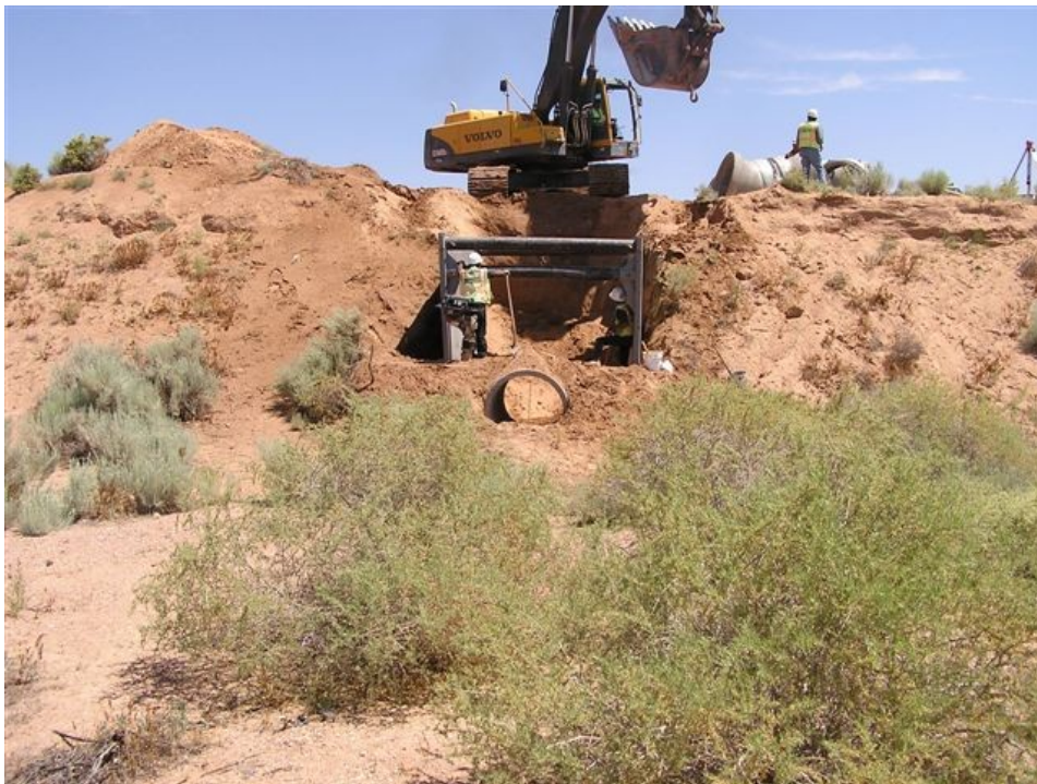
Obregon Road construction
