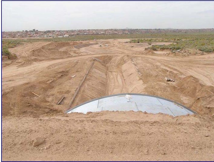
Looking south from the Multi Plate
