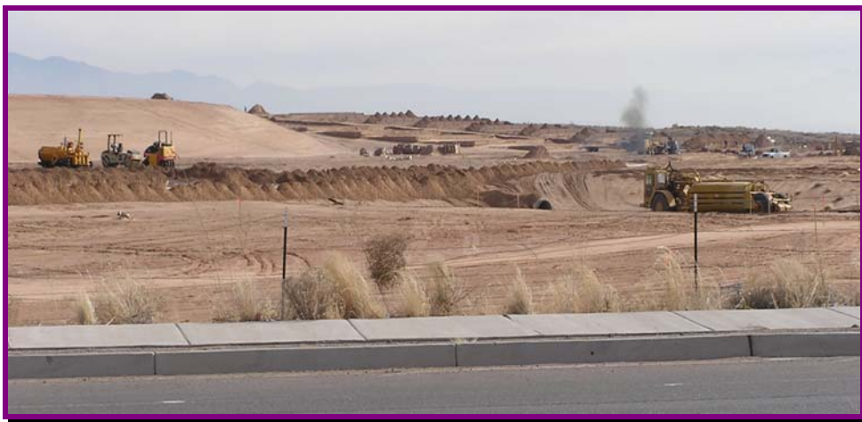
Construction in Unit 15, Northern Meadows
